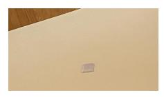
Answer to last month's trivia question: In the sanctuary, above the organ pipes, you will see this square plate. It is a reflector for the laser beam that comes from the back of the church as part of our smoke/fire alarm system for the sanctuary. If the beam is interrupted by smoke or fire, the alarm goes off.
